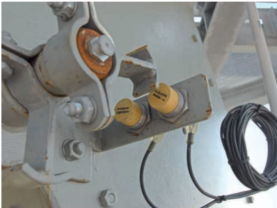
Rugged uprox sensors monitor all the butterfly valves' end positions – contact-free, wear-free and with the highest switching distances
