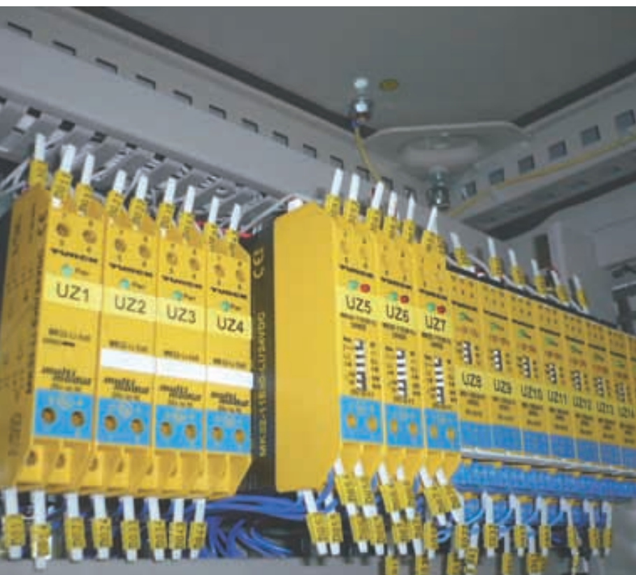
Turck interfaces are easy to install on DIN rails
