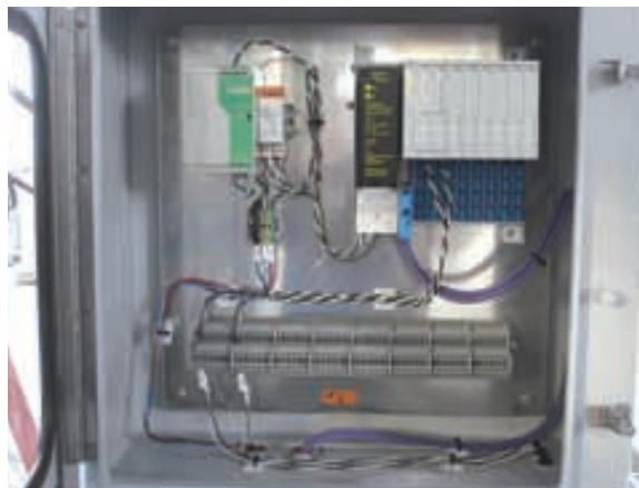
Status LEDs on gateway and I/O modules allow a simple function diagnosis of the excom station
